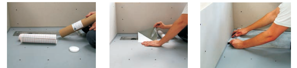
14. Remove the roll of tanking mat and lay over the drain. With the mat laid flat, peel the backing tape from one corner then back 150mm. Place the edge of the tanking mat against the inside edge of the tray and centrally over the channel. Apply enough pressure for the mat to adhere to the tray.
