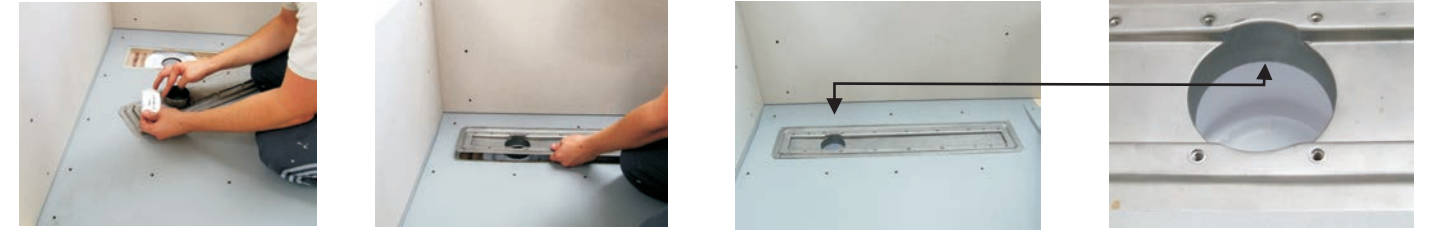
12 Open the grease that is supplied with the gully, apply half to the outer edge spigot of the main channel, set rest aside for later use. Gently push the spigot of the main channel into the gully ensuring the rubber seal inside the gully is not disturbed. The spigot of the main channel should fit flush with the bottom of the trap adaptor in the gully. With the screws provided secure the main channel to the tray. Check and test for water leakage, ensure all fittings are watertight..
