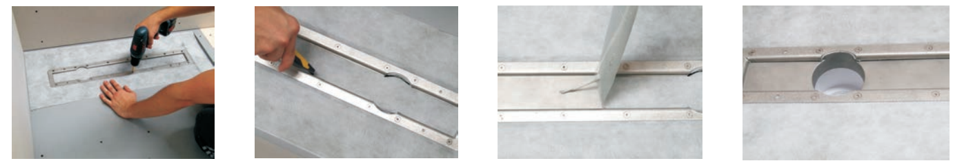
16. Position the clamping ring into the main channel and push down. Screw the clamping ring to the main channel through the tanking mat. With a sharp knife cut along the inside of the clamping ring and remove the excess tanking mat. Remove and replace the rest of the floor as necessary with 22mm waterproof chipboard or 24mm plywood to suit.
