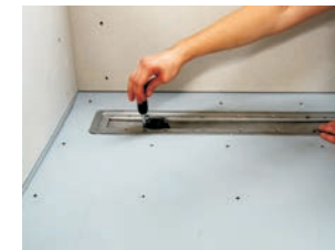
13. Remove the screws that secure the clamping ring to the main channel. Lift out the clamping ring and screws. Set aside.
