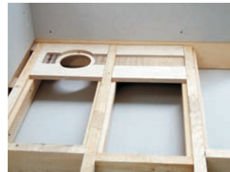
7. Lay the cut pieces of waste support on the battens ensuring they are level with the top of the joists.
