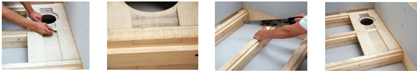
8 With a pencil, mark out the position on the joists to be notched out. Remove the waste support. Cut out a 13mm deep notch. Replace the waste supports and secure to the battens.
