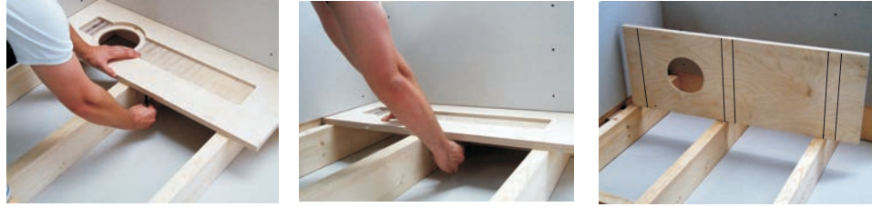
5. With a pencil, mark the position of the joists on the underside of the waste support. Cut along the marked lines, ensure the cut pieces fit between the joists.
